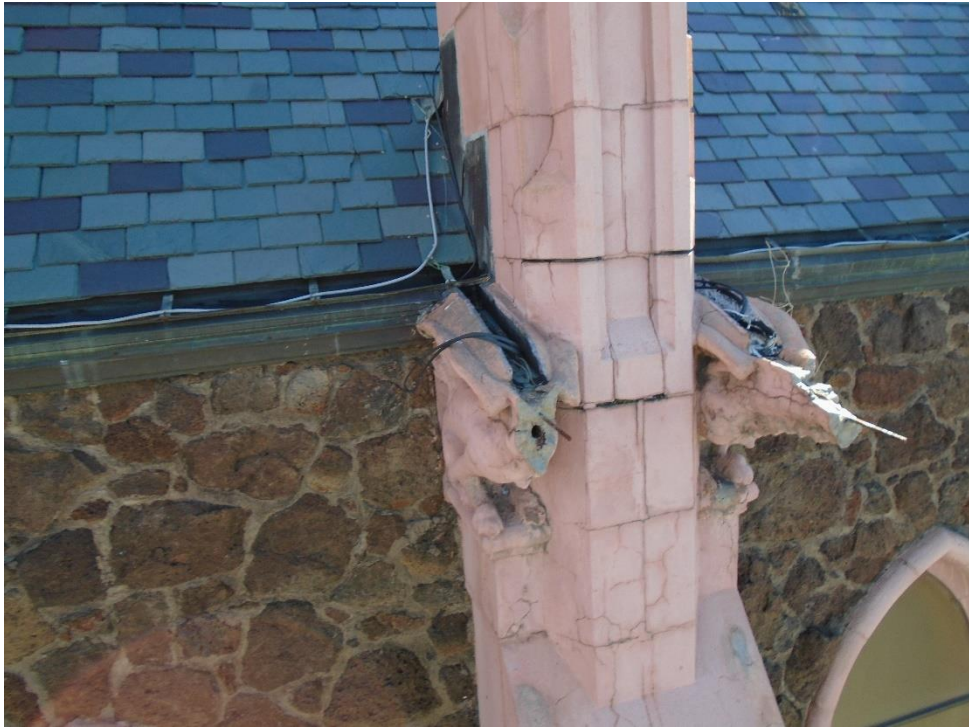
Photo 31 Heat-trace wires.
