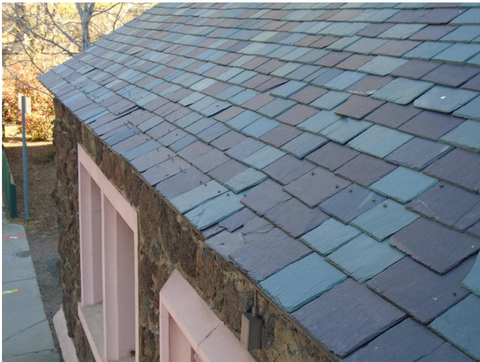
Photo 32 Steep-slope roof at rear of church.
