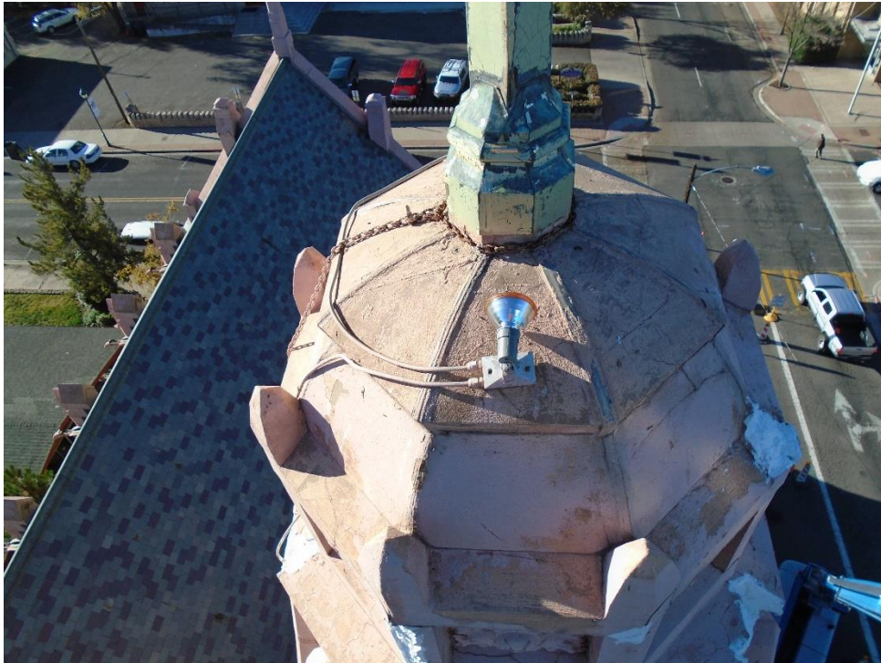
Photo 77 Roof of cupola.
